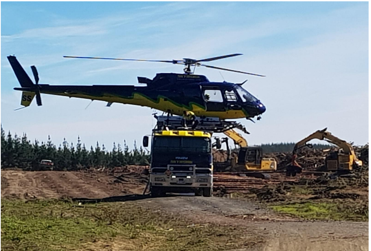
Preparing to spray area for forestry planting
